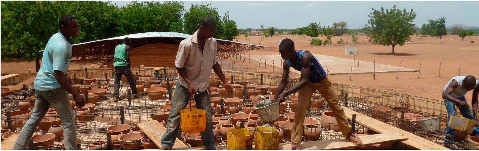
108. The claypots being used in construction
