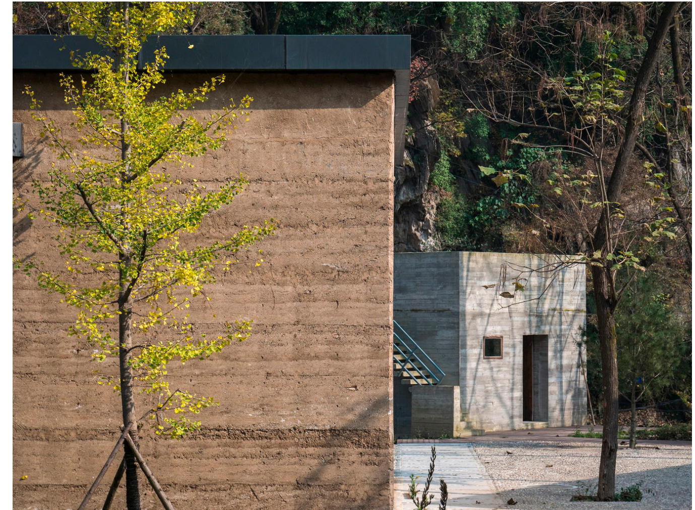
88. Use of rammed earth allows for the use of local materials, it is the quintessential 'local' material since it often comes directly from the site itself.
