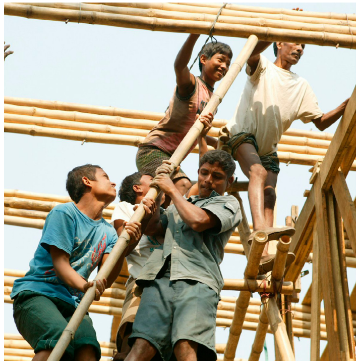
94. People lifting bamboo poles, since cranes are not always available
