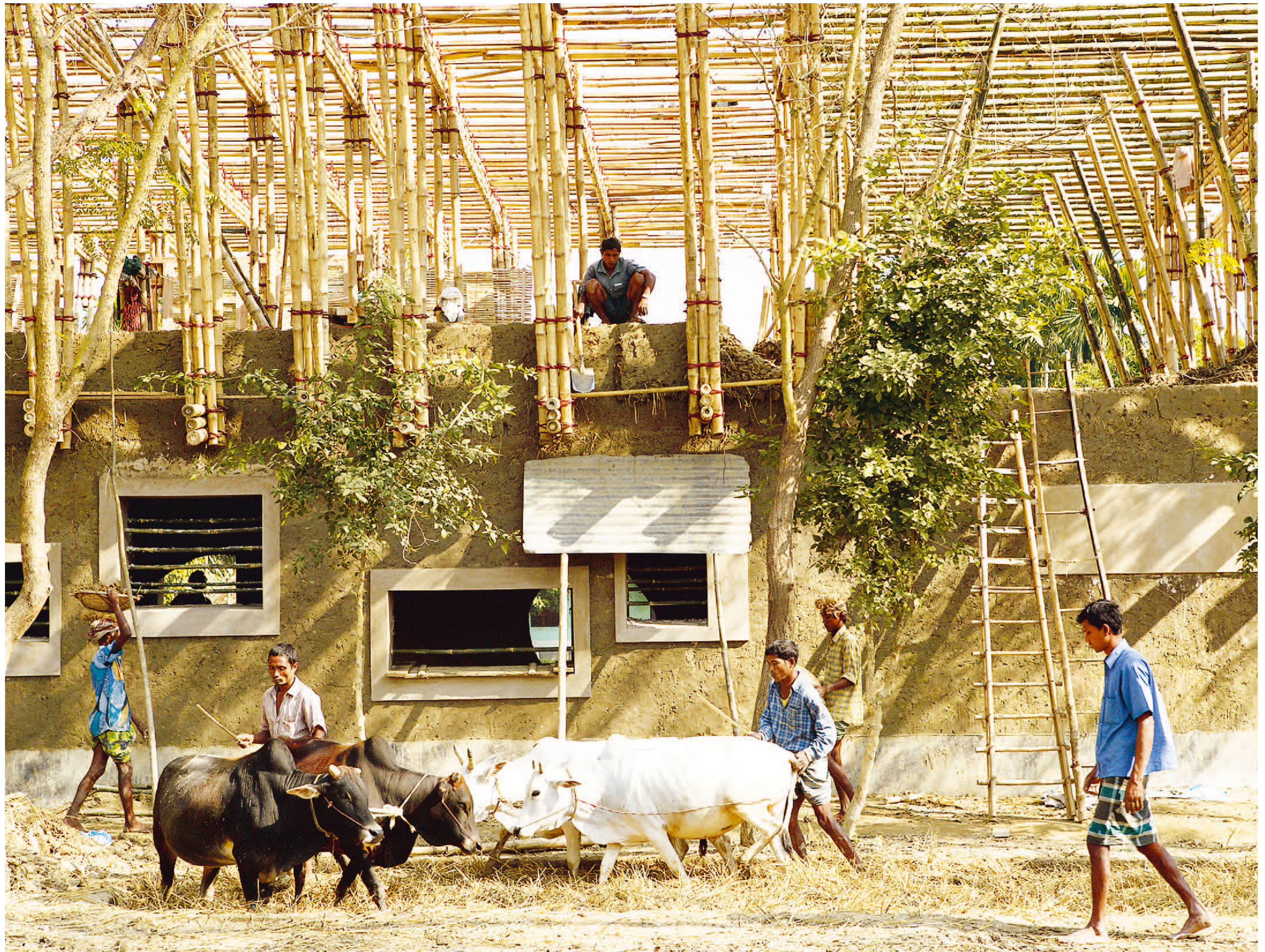
97. Animals being used to mix concrete
